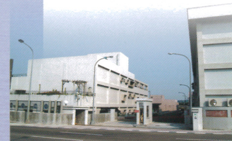
行政大樓 Administration Building
