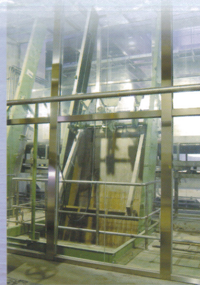
粗欄污柵 Coarse Bar Screen
